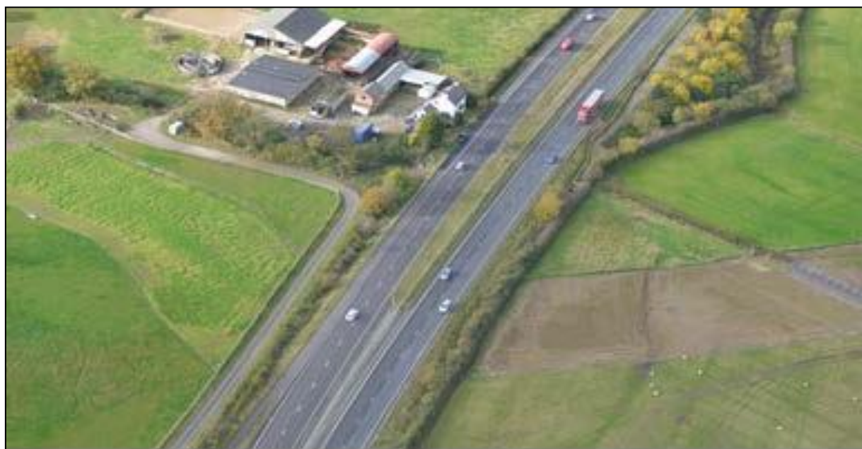
Figure 1.15: Cable corridor during restoration example (RWE renewables UK Ltd)
